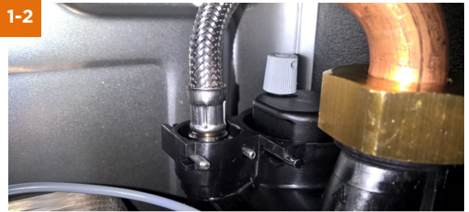
Flue system is all connected, auto air vent in the boiler is open.
